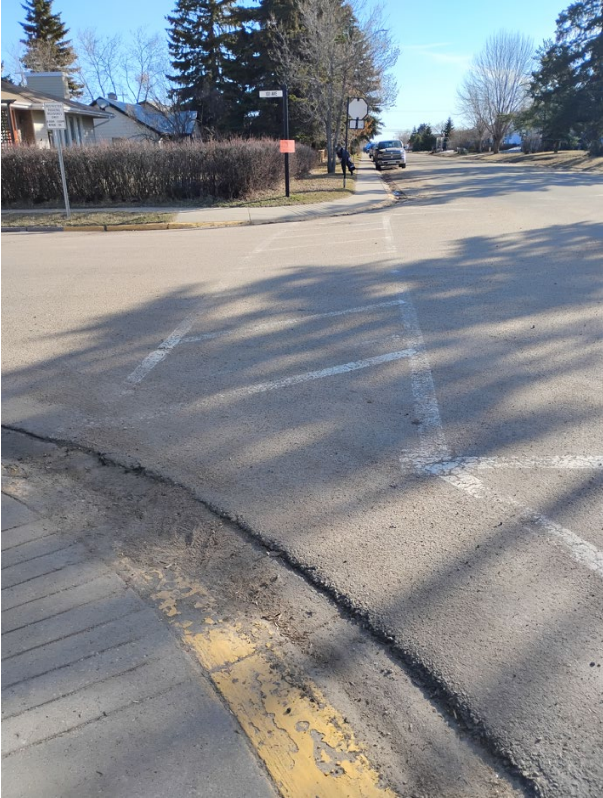
#21 - 104 Street & 100 Avenue (RF Staples School, North Side)
