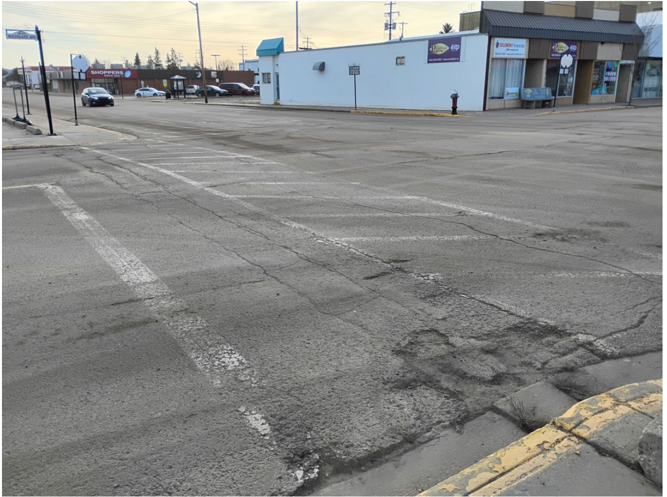
#3- 107 Street & 100 Avenue – North Side
