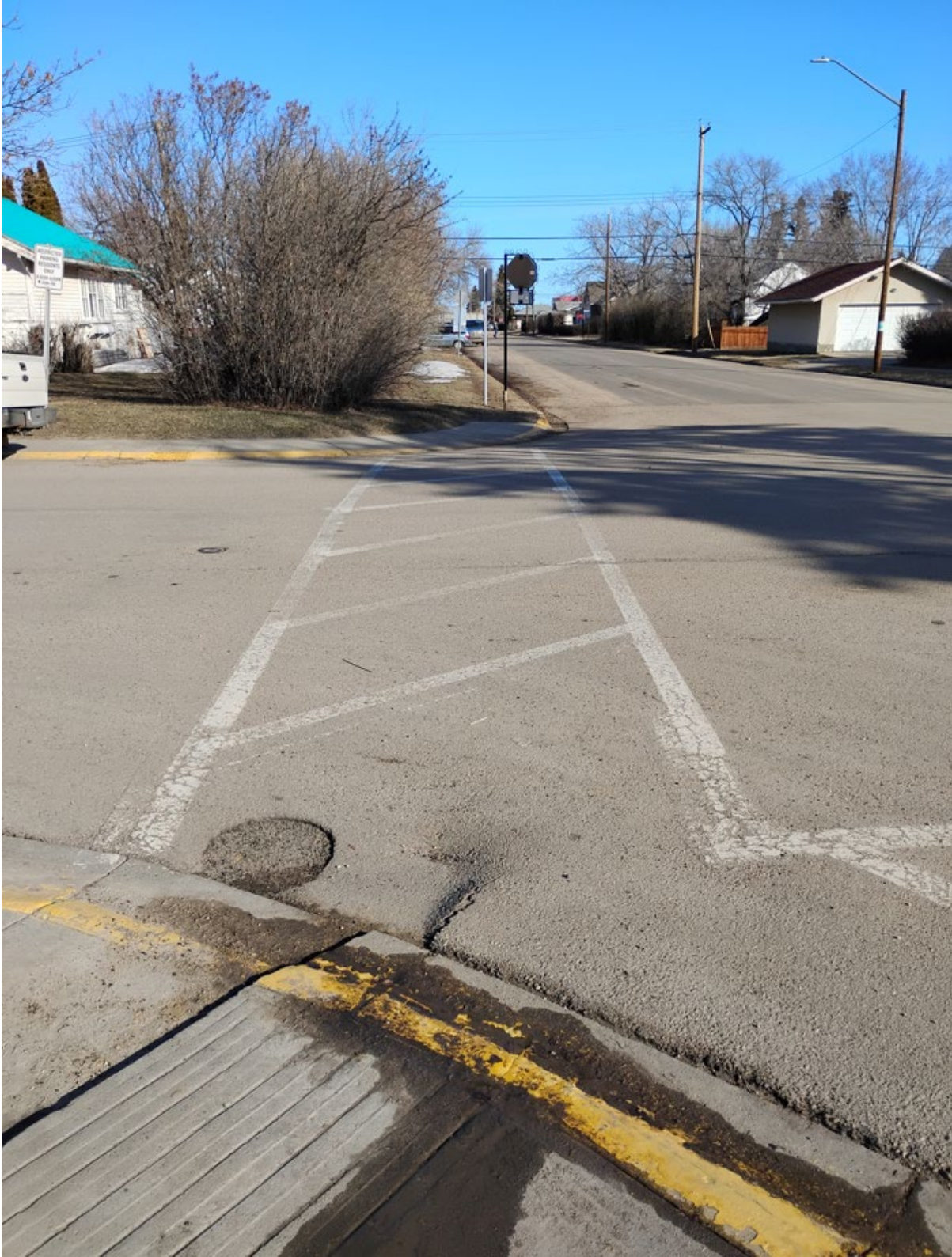
#20 - 104 Street & 100 Avenue (RF Staples School, West Side)
