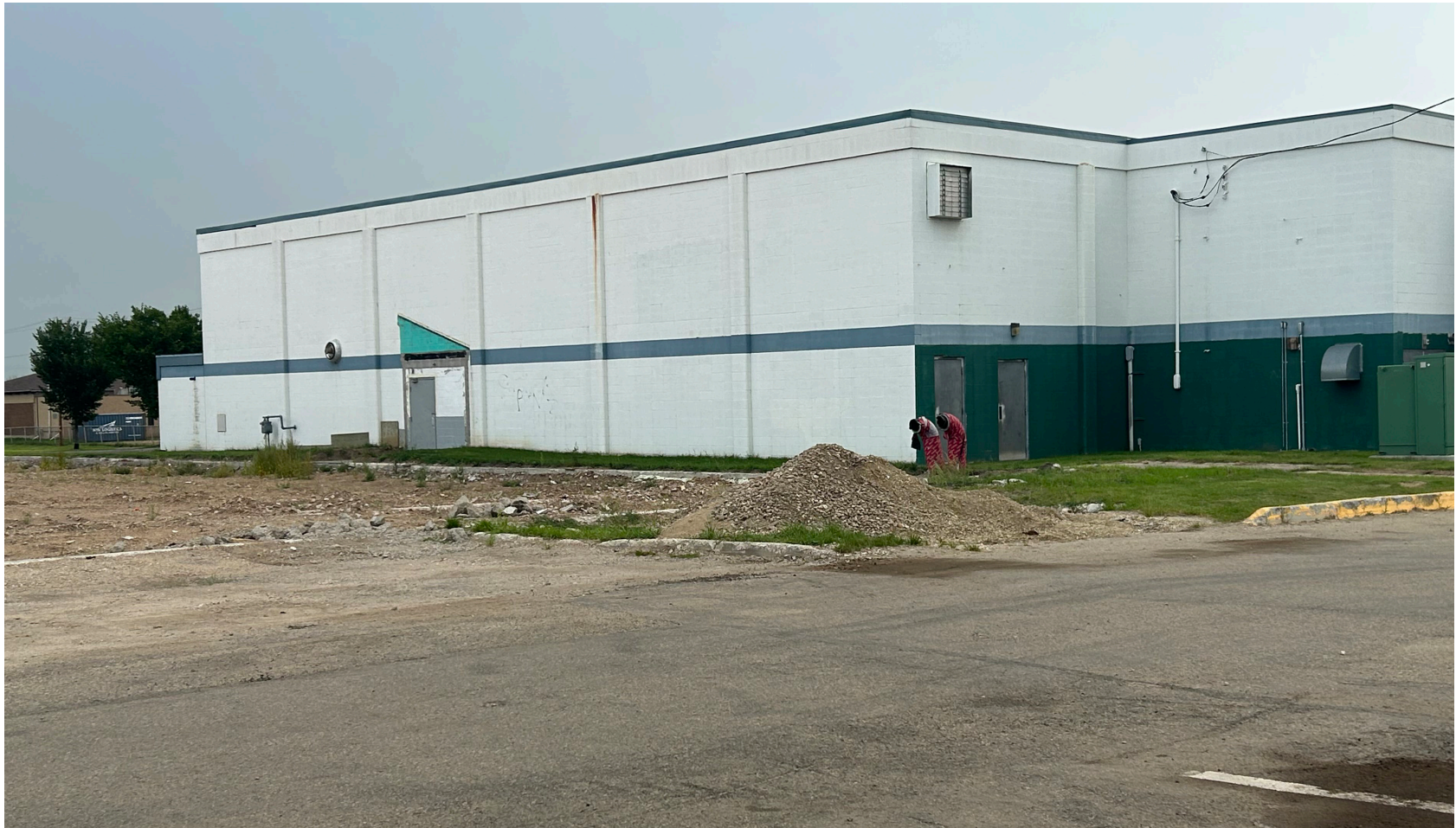
Current Facade - Rotary Spirit Centre, Westlock
